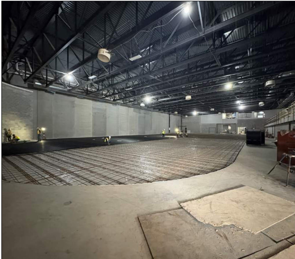
Auxiliary Ice Subgrade Preparations
