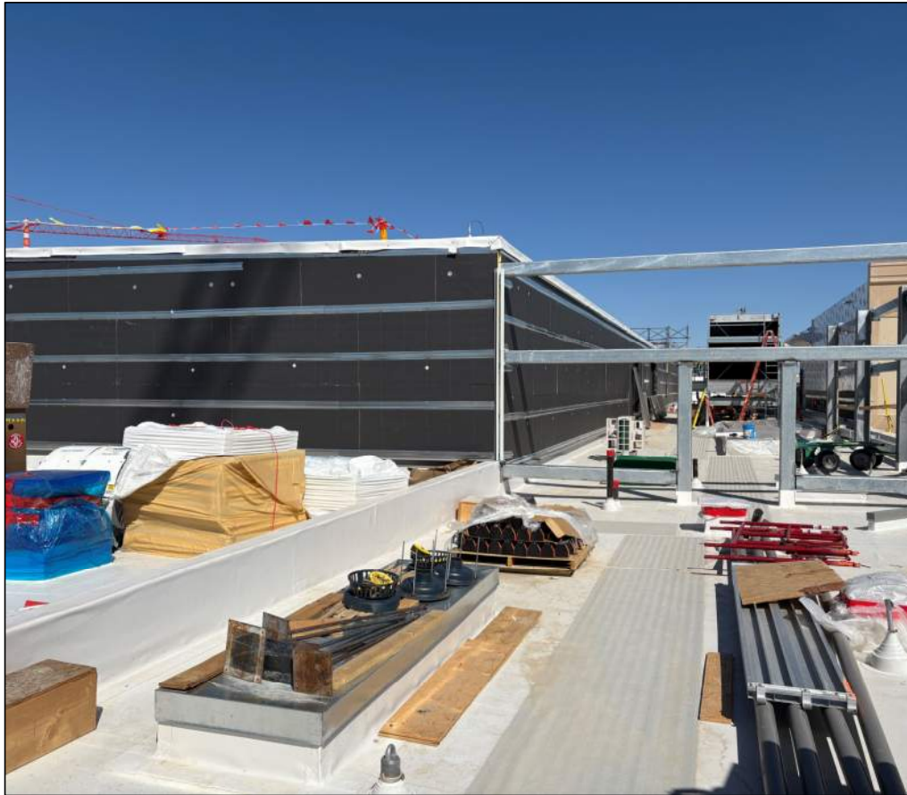
Main Arena South Low Roof Exterior Sheathing
