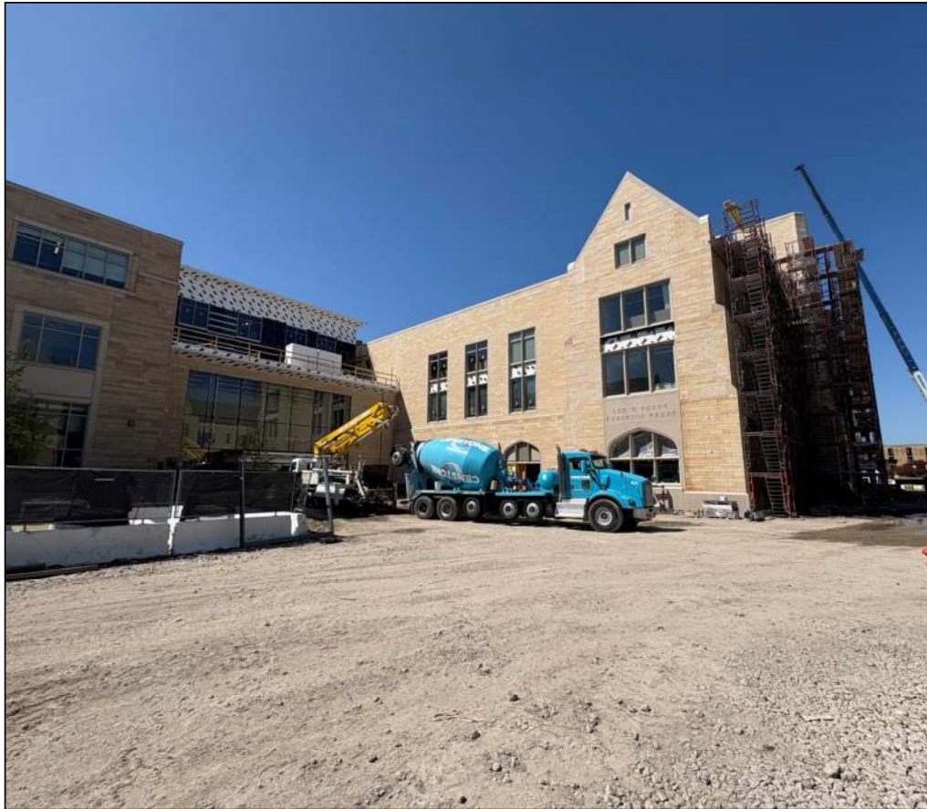
Student Entry Exterior Elevation Sheathing Installation In Preparation for Metal Panels
