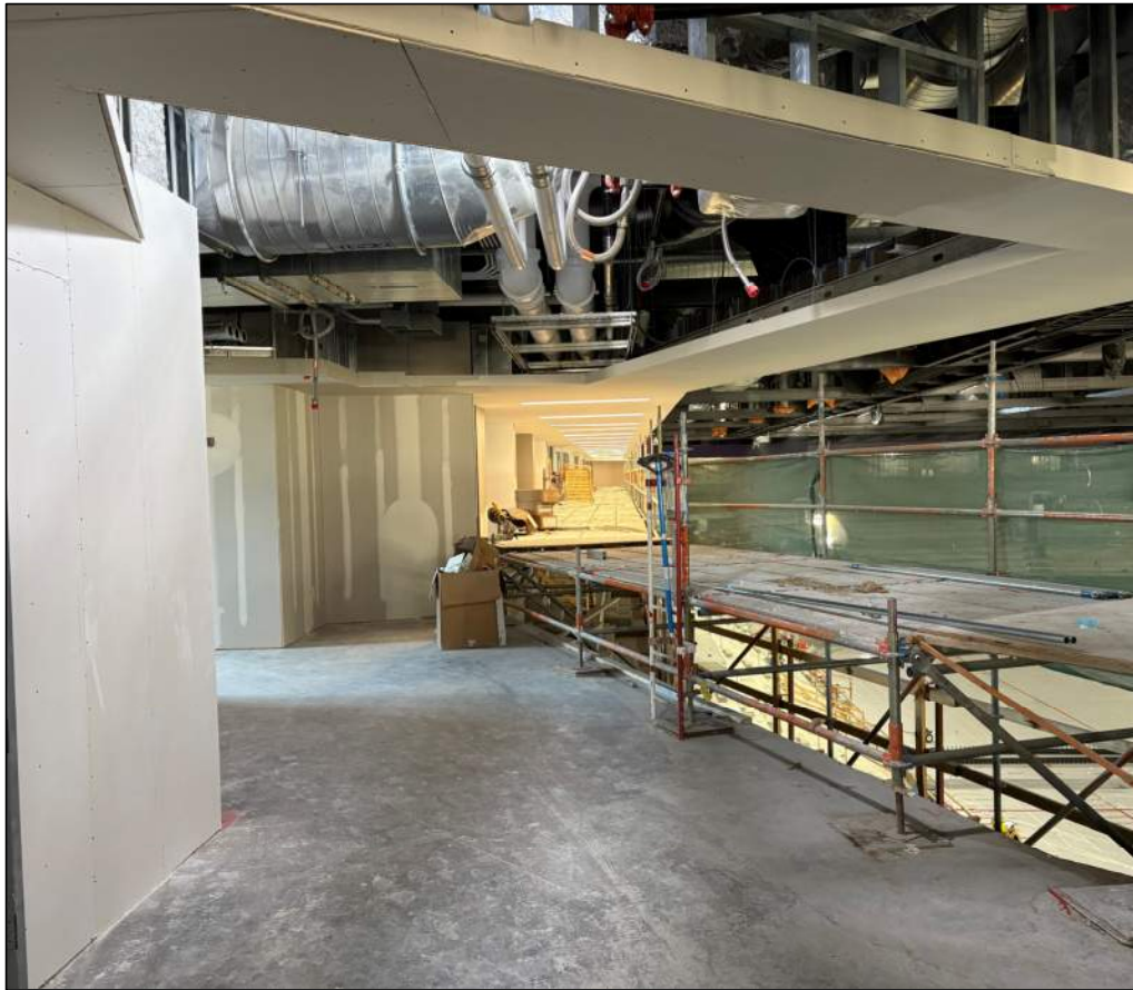
Main Arena Club Level Soffit Framing
