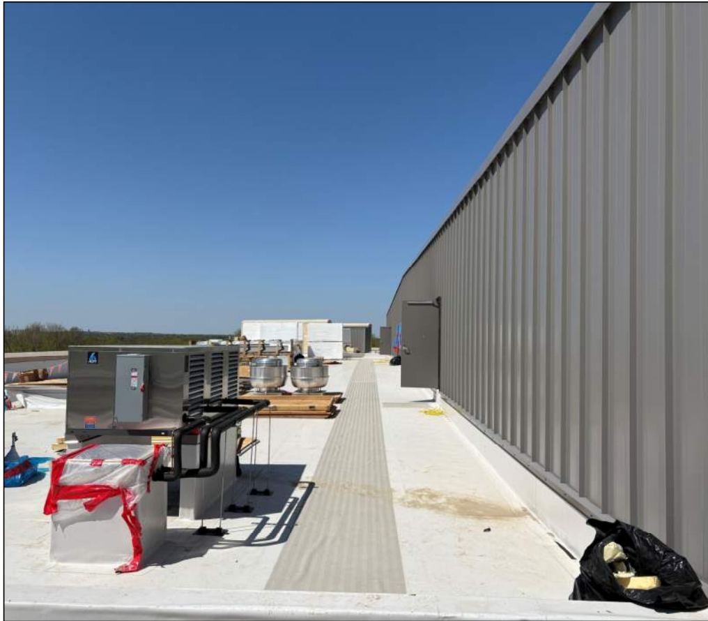
Main Arena South Low Roof Exterior Metal Panel Installation
