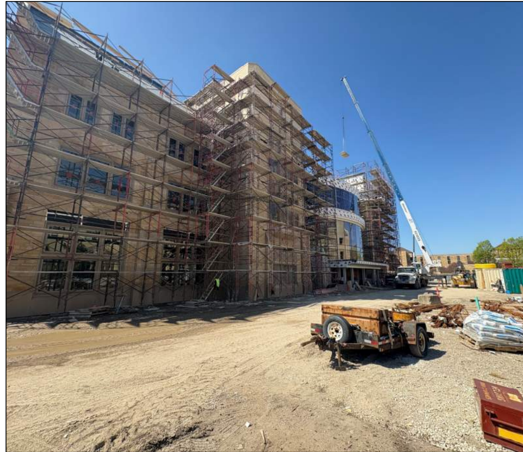
Main Arena North Exterior Elevation Stone and Glazing Installation
