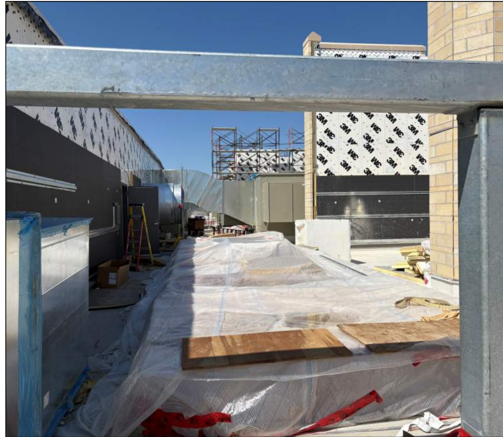
Exterior Sheathing and Metal Panel Installation at Main Arena North Low Roof
