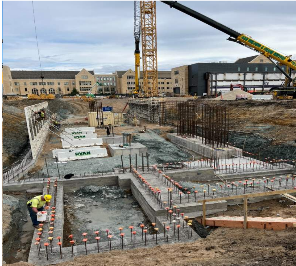
Basement foundation wall installation
