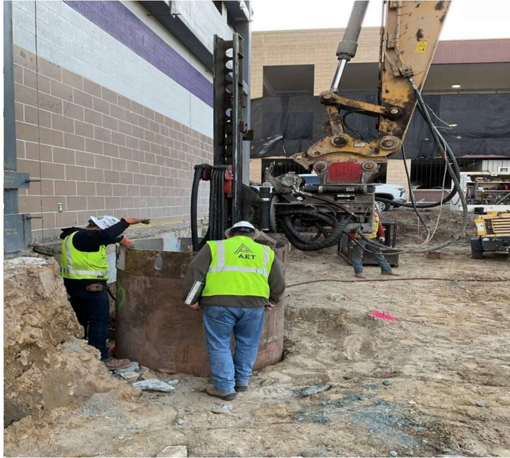
Drilled piers installation
