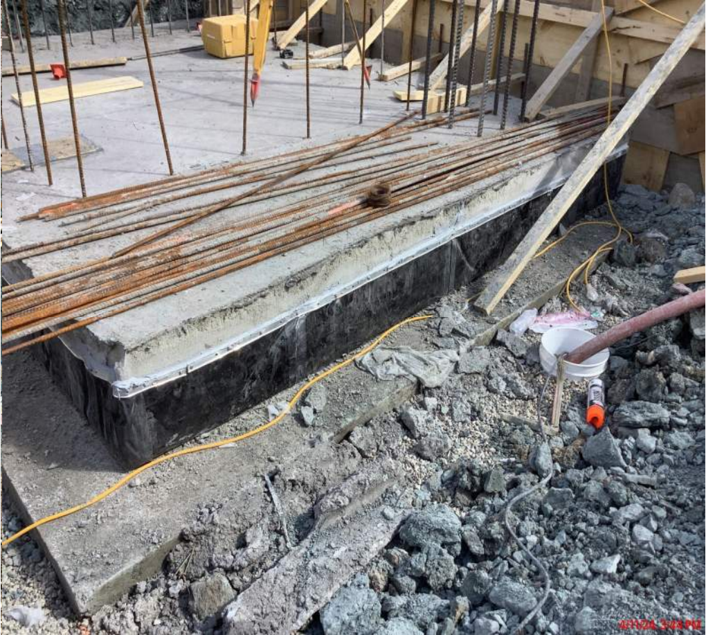
Waterproofing for elevator slab
