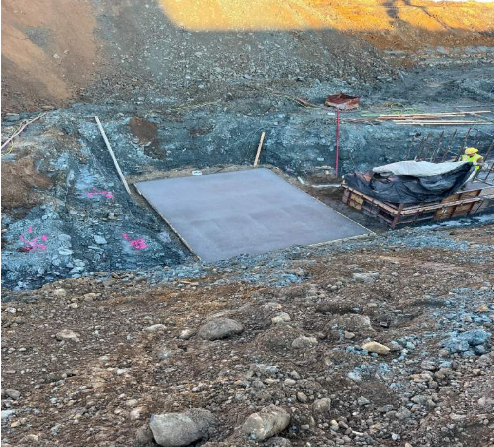
Poured elevator pad S05
