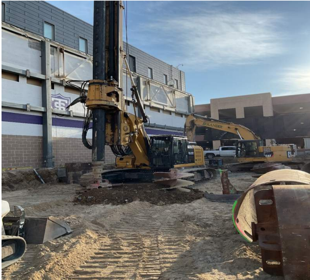
Drilled piers installation
