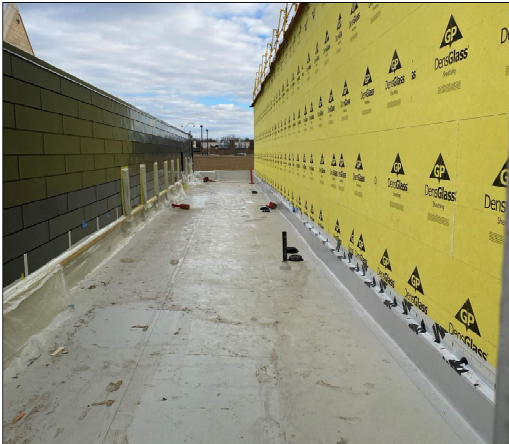
Roof and Exterior Sheathing Installation – Club Level North
