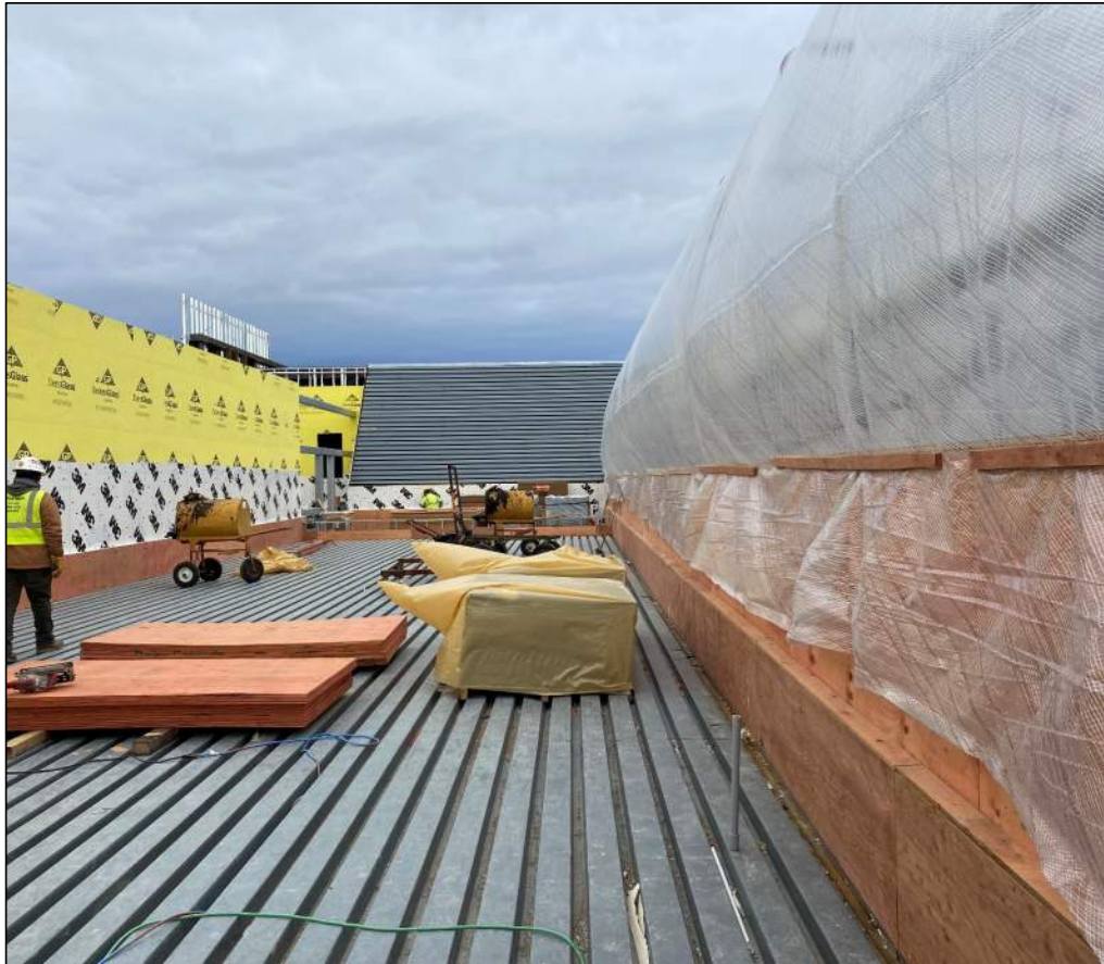
Exterior Wall Sheathing and Metal Deck Installation – Concourse Level
