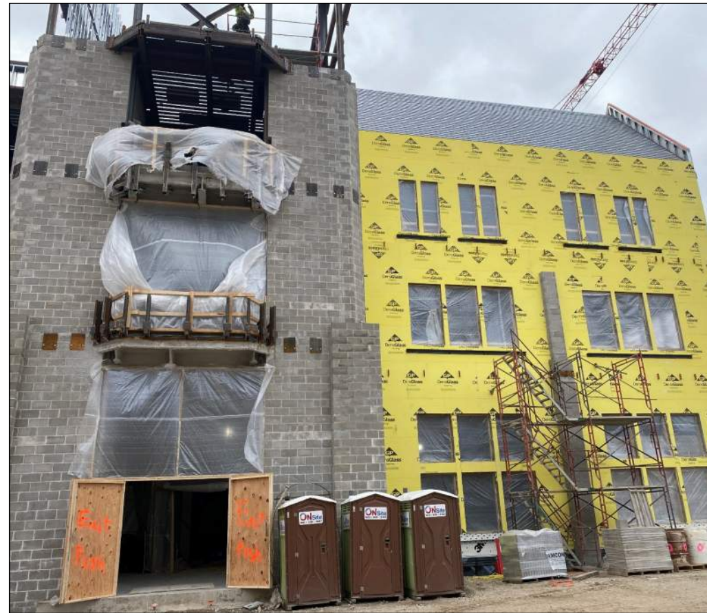
Exterior Sheathing and Roof Decking - North
