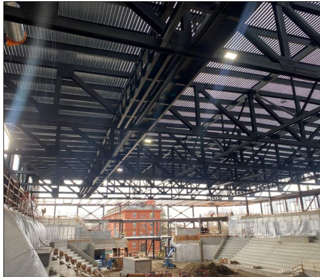
Roof Deck Installation – Main Arena
