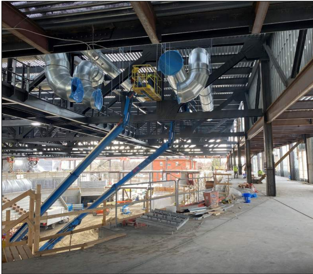
Main Arena HVAC Pipe Installation – Club Level
