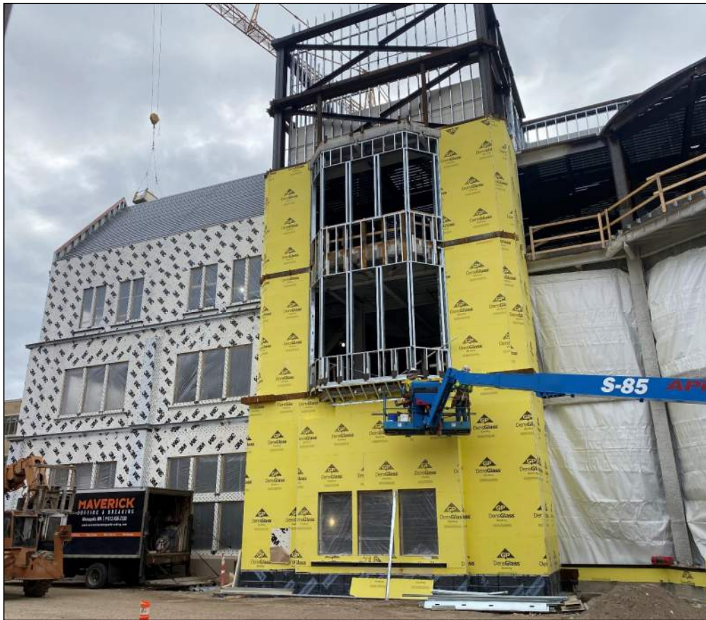
Exterior Framing, Roof Decking, Sheathing and Weather Barrier Installation - North
