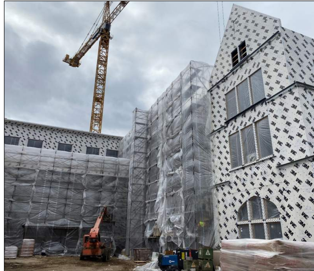
Weather Resistant Barrier Installation – Northeast Side
