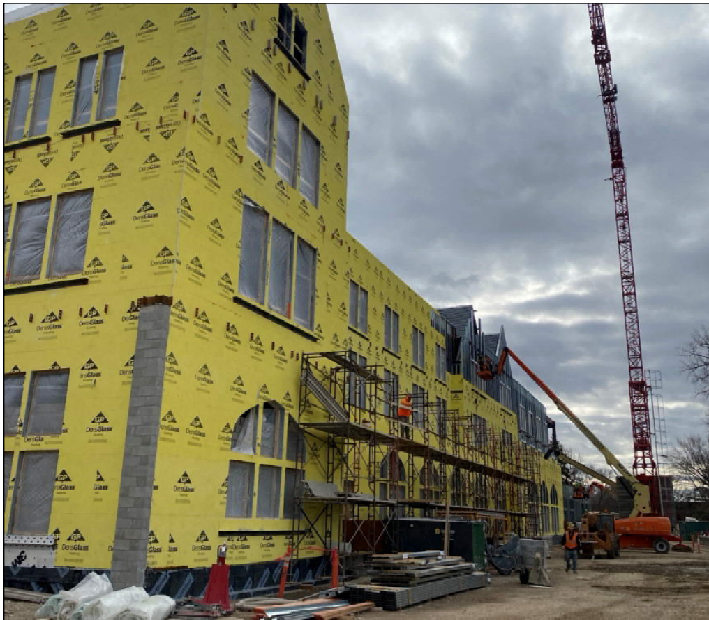
Exterior Wall Framing and Sheathing - West
