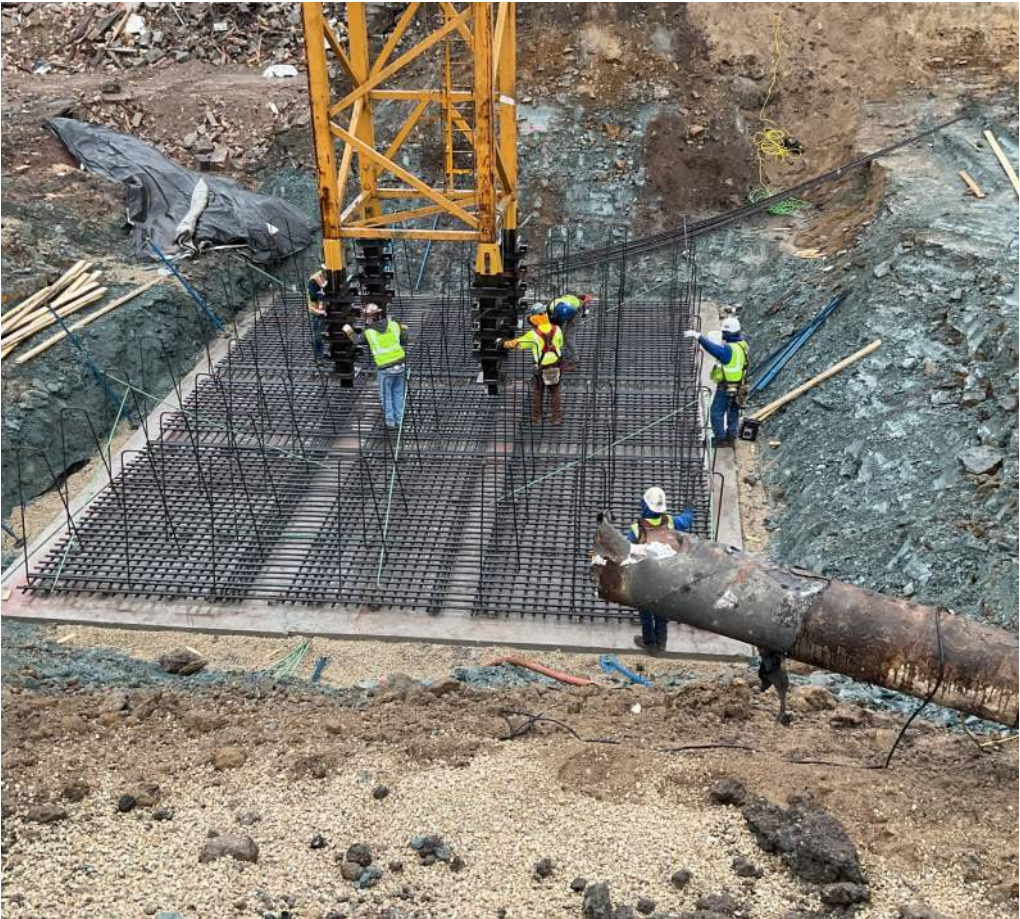
Reinforcing install for crane pad
