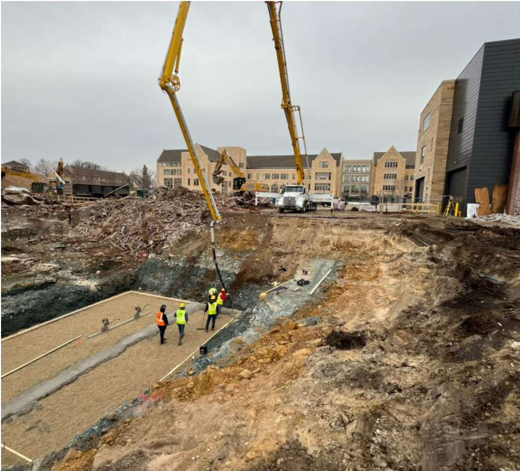
Working slab for crane pad being poured
