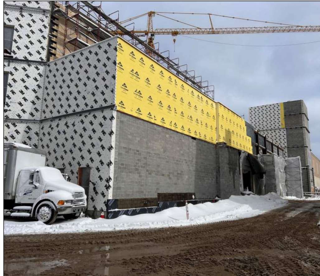
Main Arena South Elevation Exterior Stone and Sheathing Installation
