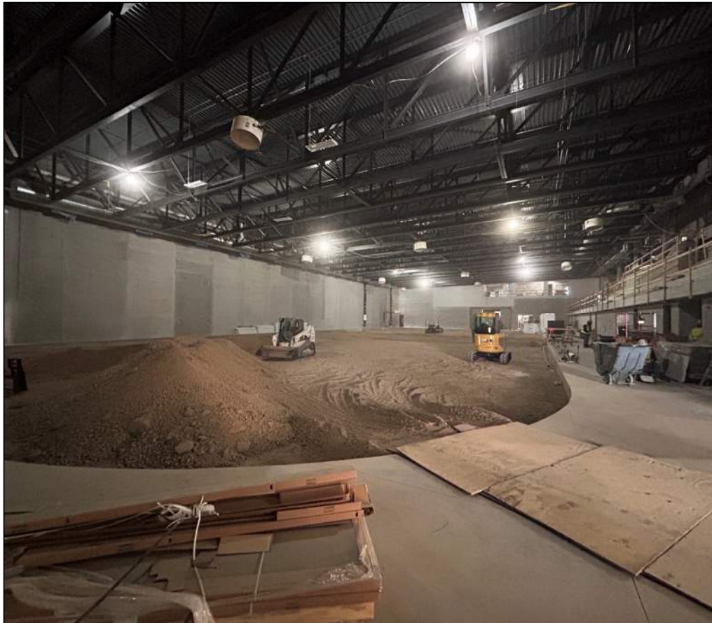
Auxiliary Ice Subgrade Preparations
