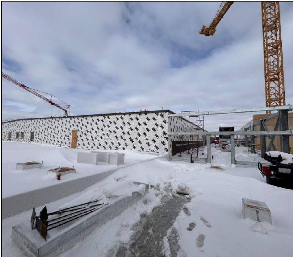
Main Arena South Low Roof Exterior Sheathing
