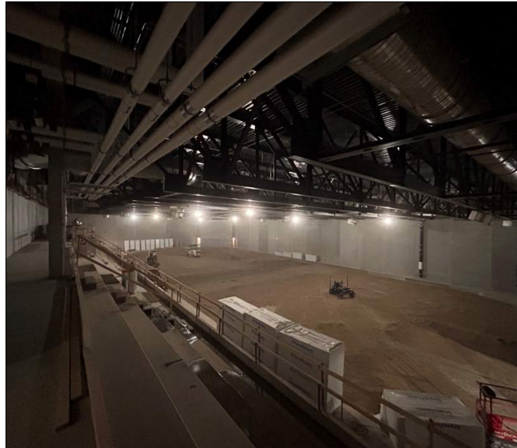
Auxiliary Ice Subgrade Preparations
