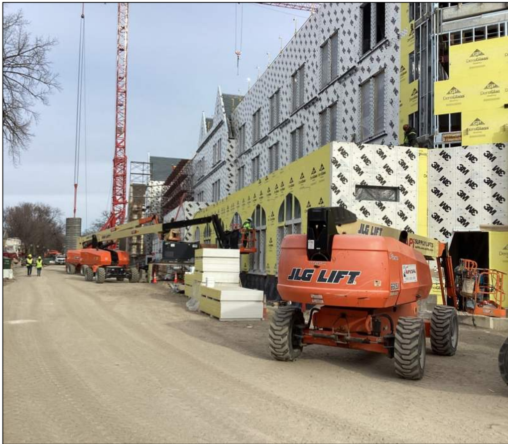
Exterior Framing, Roof Decking, Sheathing and Weather Barrier Installation - West
