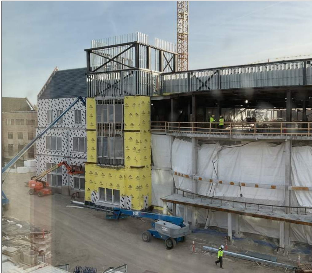
Main Arena North Exterior Elevation Framing and Sheathing
