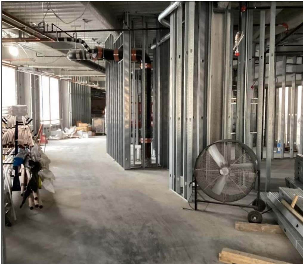
Interior Framing Northeast Concourse Level
