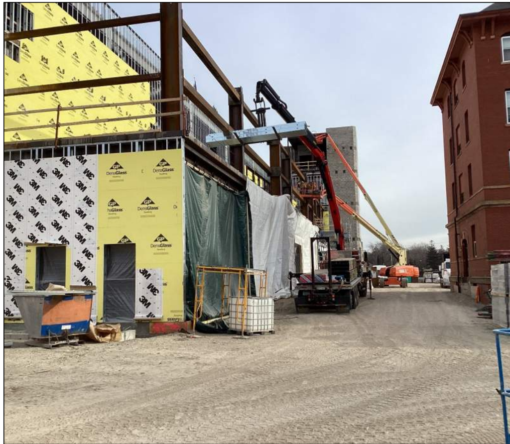
Exterior Sheathing and Roof Decking - South
