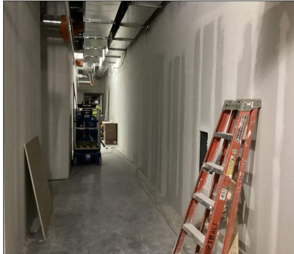
Interior Gyp Framing at Soccer Corridor
