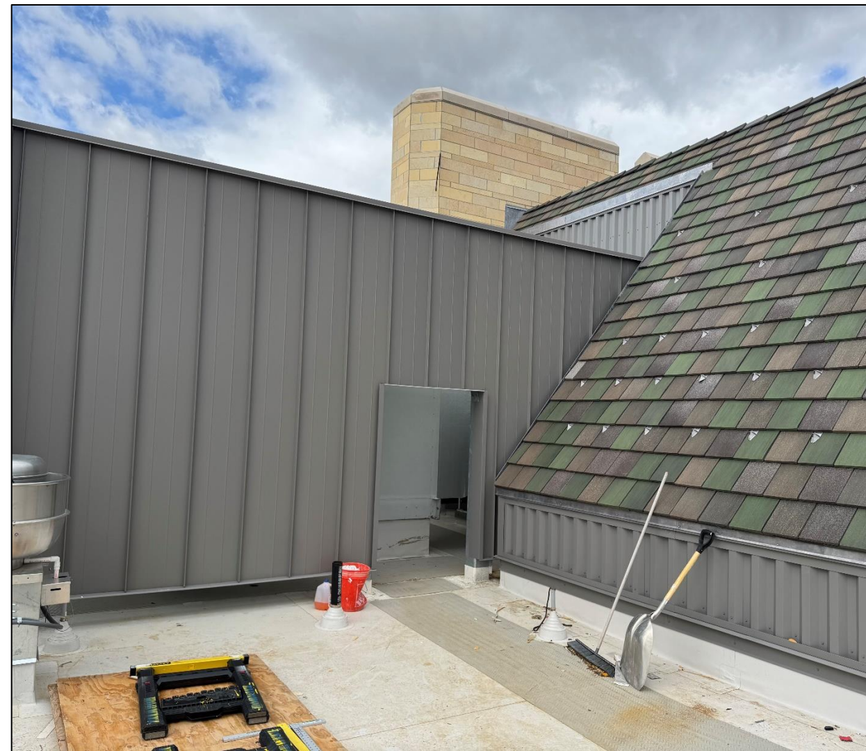
Main Arena North Roof Metal Panel Completion
